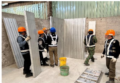
Replacement of wooden molds with 300-times reusable aluminum molds
